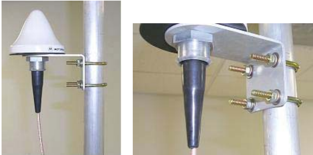
Figure 9: Detail of GPS antenna mounting
